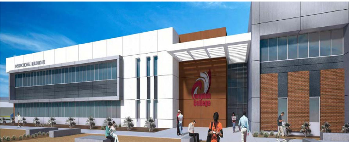
INSTRUCTIONAL BUILDING 2 $25.6 million, new construction Est. Completion: Fall 2021
